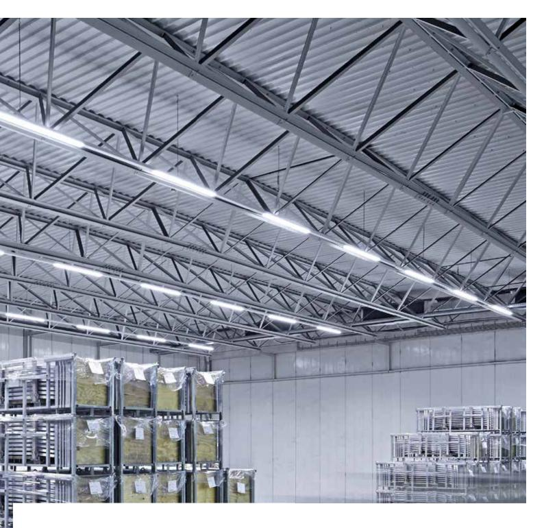
Warehouses are a world of their own – large, windowless halls with high shelving constructions and relatively narrow aisles where workers need to move quickly and safely. Ideal lighting solutions are high-performance and durable luminaires with narrow or narrow-wide distribution reflectors and high levels of glare reduction. Optimum visual conditions must exist when looking up towards the hall ceiling as well, e.g. when sorting goods at high heights with forklift trucks.
